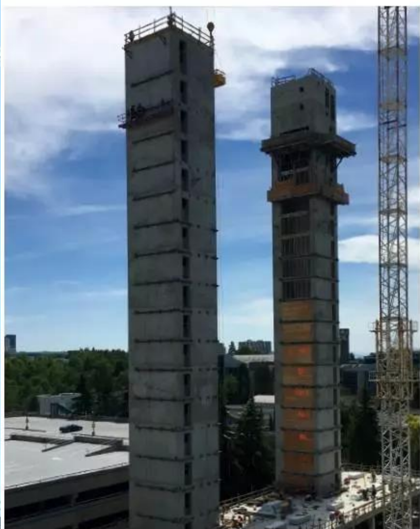
微信号: canadawoodchina Construction of concrete cores (June 2016)
